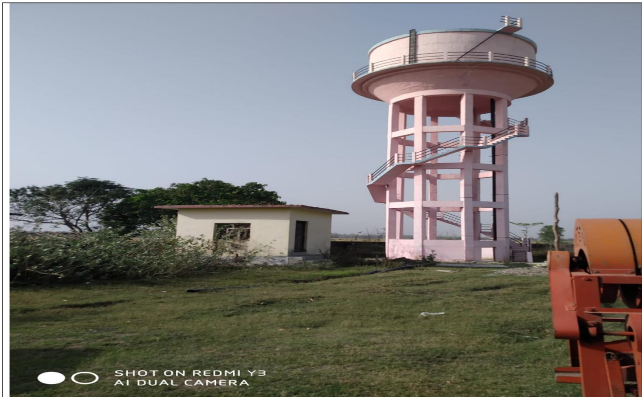
Existing structures at the LokhariWSS sub-project, OHT premises
