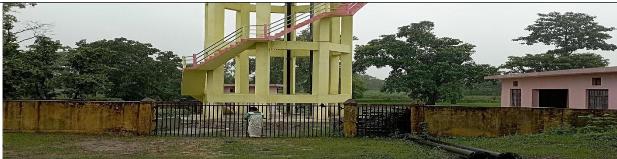
9. Complete Boundary Wall and Gate
