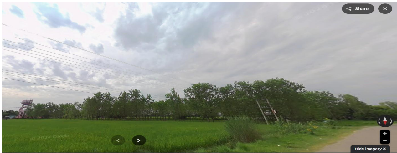
12. Google Map showing the both existing OHT premises and Transfoemer
